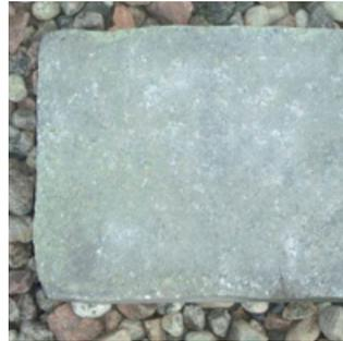
Because efflorescence occurs when mineral salts that are always present in concrete products migrate to the surface, once these salts are exhausted, efflorescence will stop. In most cases, it will simply go away.
